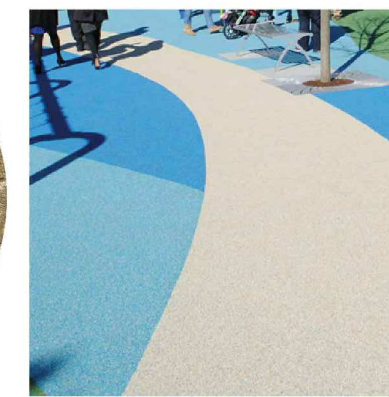
PLAYGROUND PROTECTIVE SURFACING POURED-IN-PLACE RUBBER COLOR: VARIES
