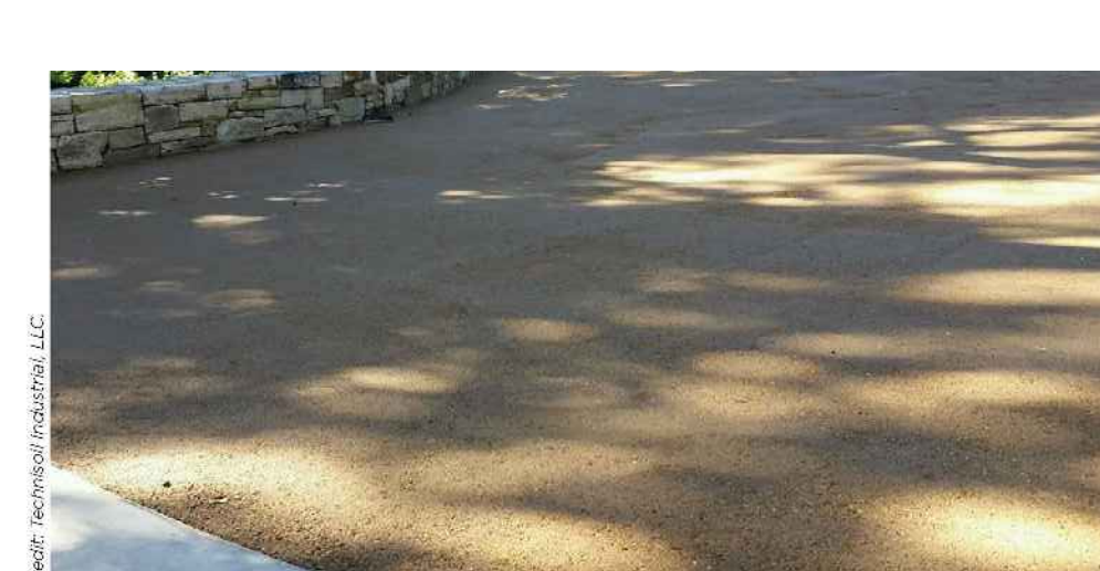
STONE FINES PAVING
