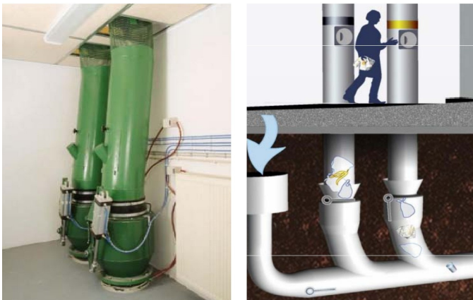
Diagram 1.5.2.2 – Example of Pneumatic Waste System Valve Room
