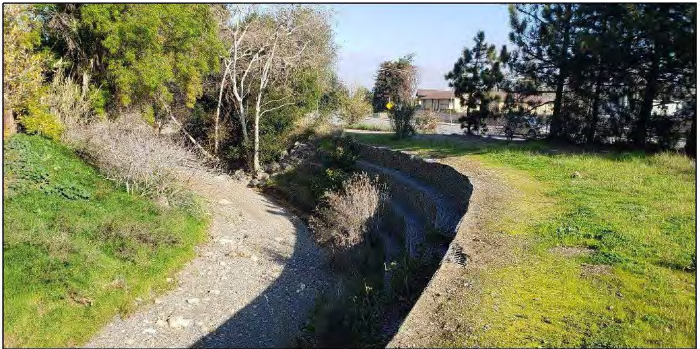
Photo 6. Viewing northeast along the armored portion of the creek channel
