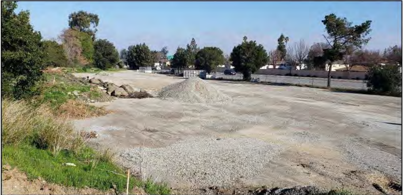
Photo 3. Viewing northeast across the site from atop the berms along Saratoga Creek.
